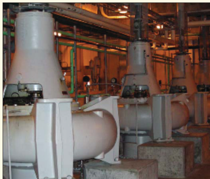
Effluent pumps, sealed with 8.00 inch (200 mm) diameter split seals, have been in service for over 12 years.
